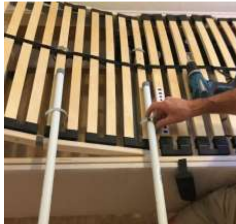
Slip the grab handle through the Jubilee Clips
